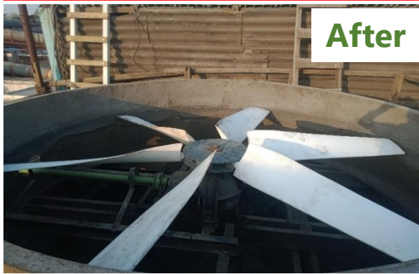
Aerodynamic Design Fan Blades for ER Cooling Tower 4 & 6
